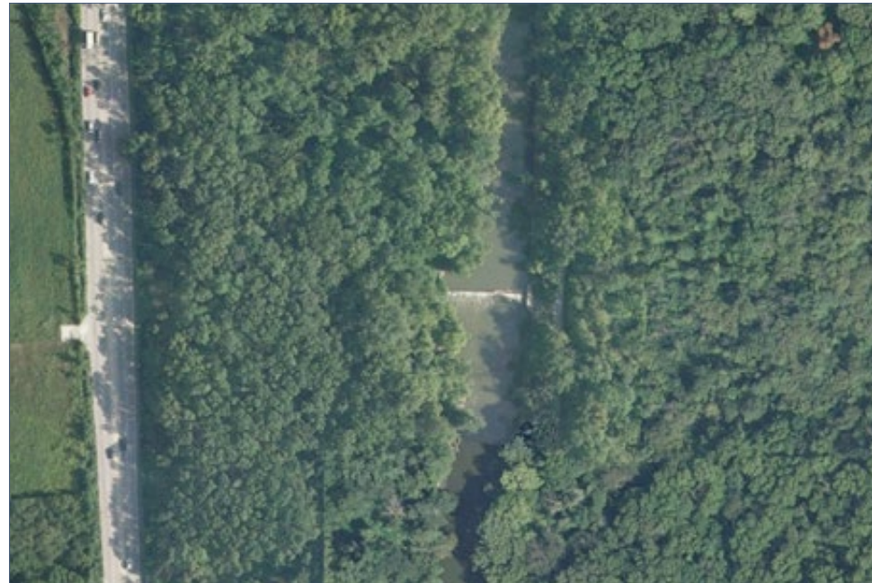
FIGURE 2.8-5 | Armitage Dam before removal.
