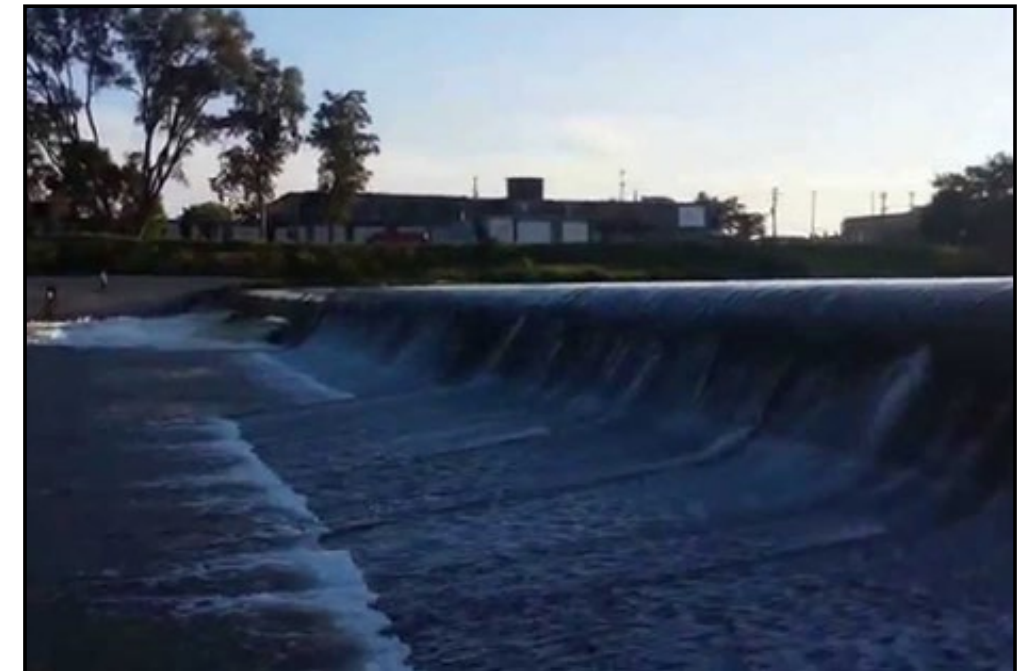
FIGURE 4.6-4 | Troy low-head Dam
