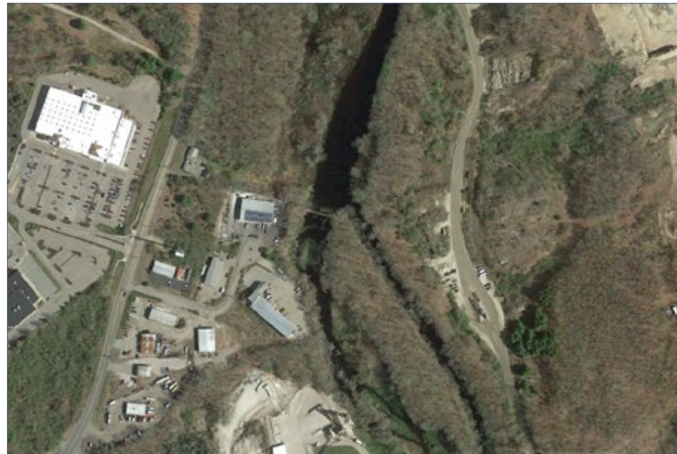
FIGURE 2.8-9 | White Rock Dam before removal, May 2015
