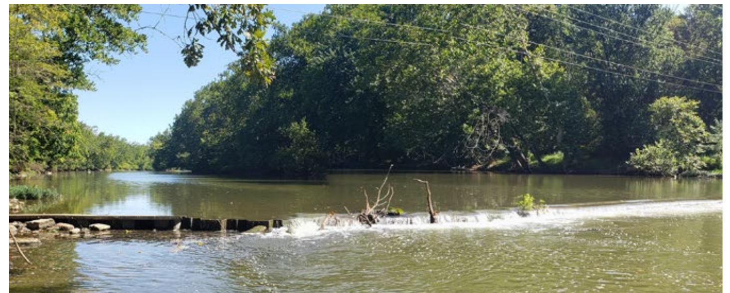
FIGURE 6.3-3 | Existing Condition of the Piqua Water Works Dam and Backwater.
