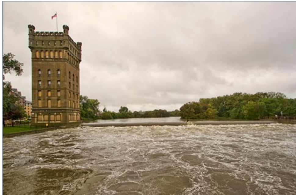
FIGURE 2.8-3 | Hofmann Dam before removal, April 7, 2017
