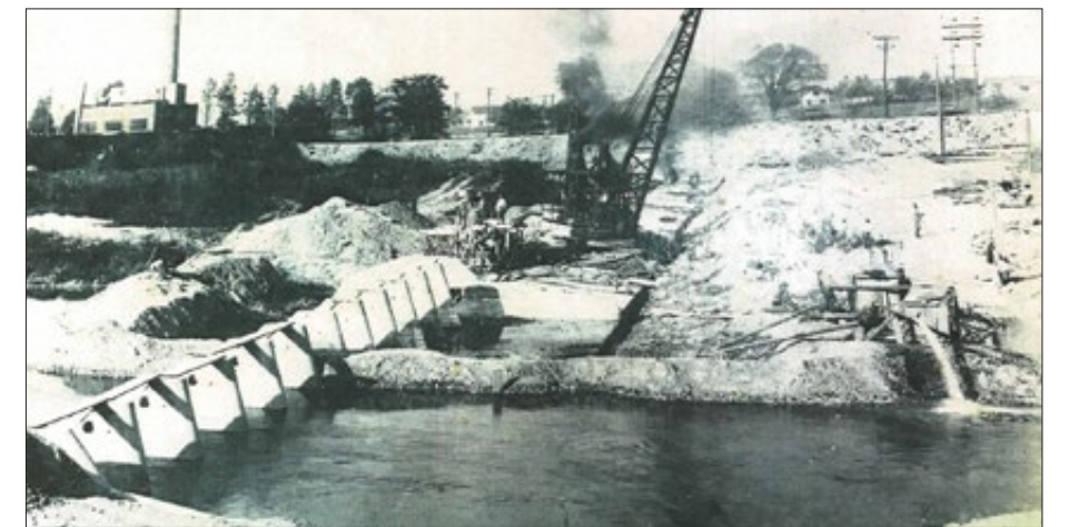
FIGURE 4.5-3 | Construction of Troy low-head dam in present-day location. ca. 1923.
