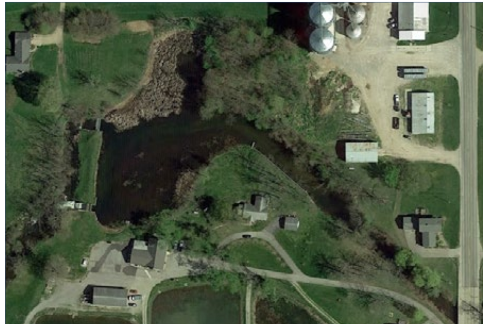
FIGURE 2.8-21 | Fawn River Fish Hatchery Dam before removal. April 23, 2017
