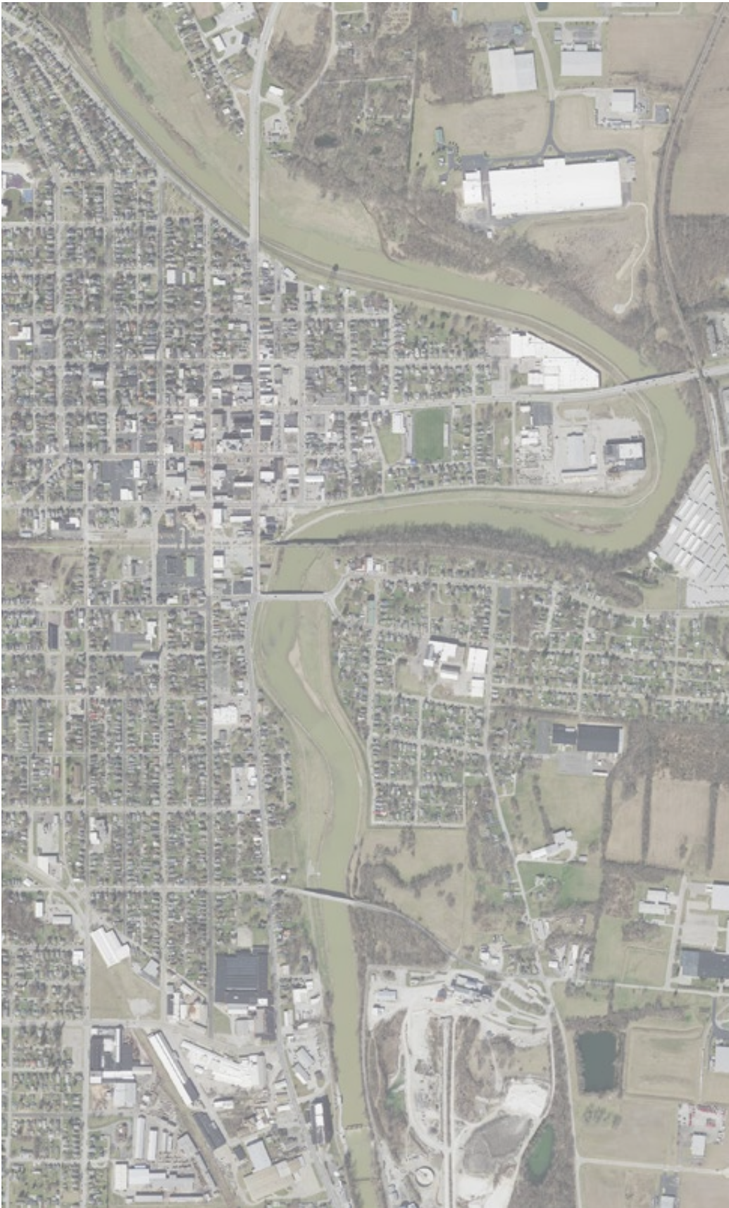
FIGURE 7.2-1 | Existing Conditions of the Piqua Dam Backwater
