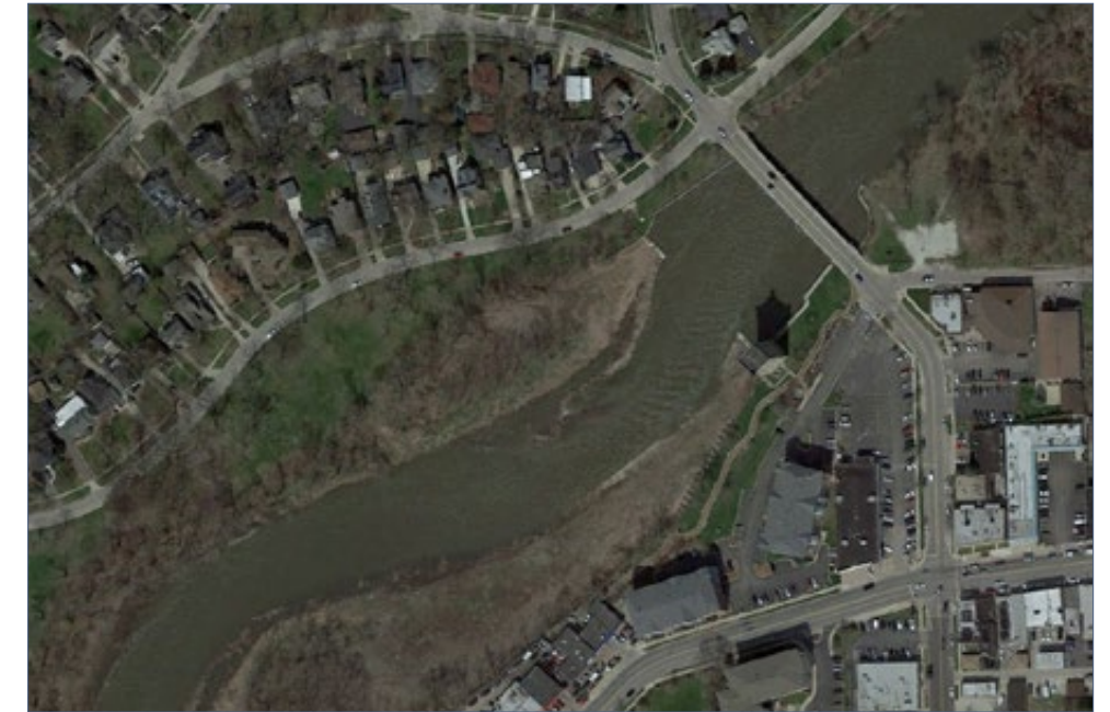
FIGURE 2.8-2 | Hofmann Dam after removal
