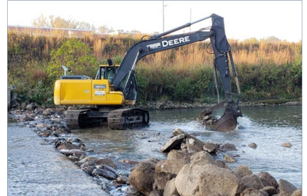
FIGURE 2.8-42 | An excavator is used to construct the riffle. October 10, 2019.
