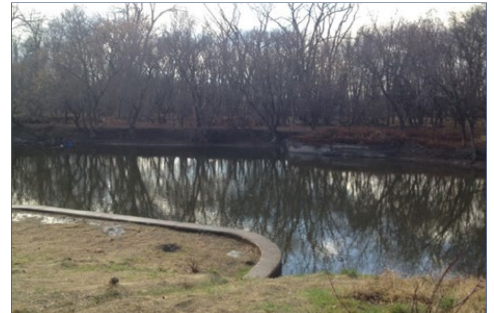
FIGURE 2.8-8 | Armitage Dam after removal.
