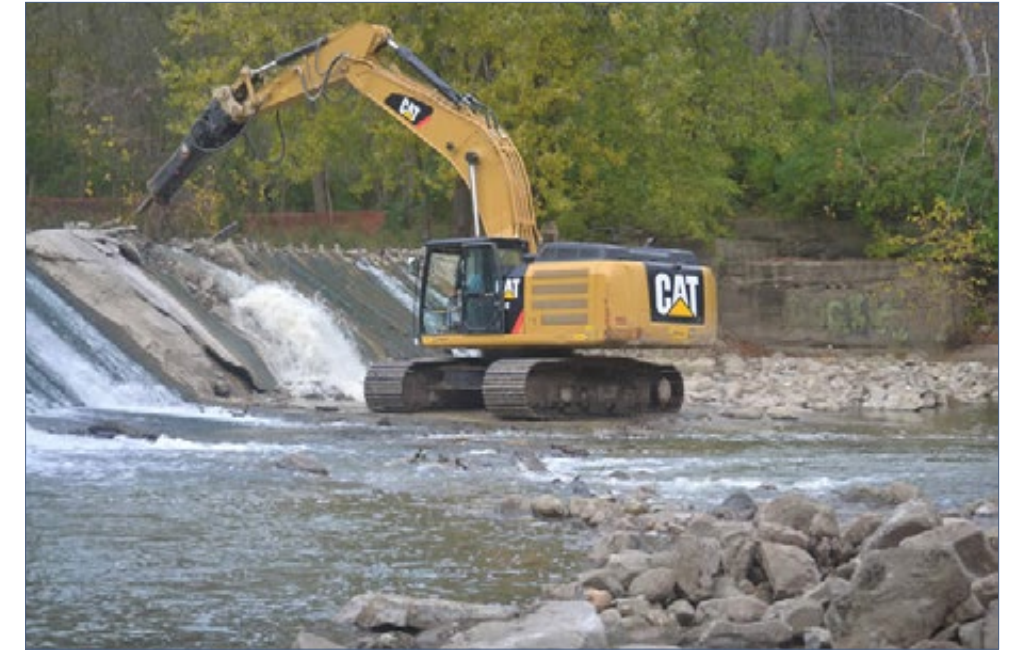
FIGURE 2.8-30 | The West Milton Dam is breached, or lowered 3 feet, to gradually release silt and save mussels upstream.
