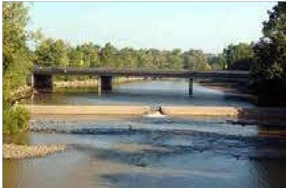
FIGURE 2.8-47 | Central Avenue Dam before removal, 2007
