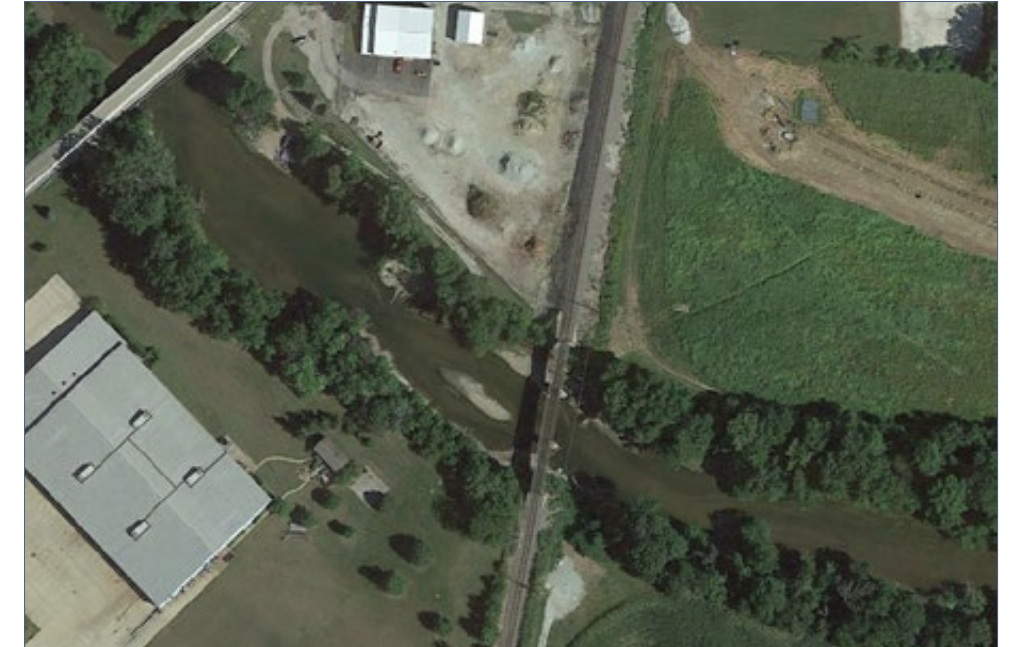
FIGURE 2.8-18 | North Manchester Dam after removal, August 23, 2013
