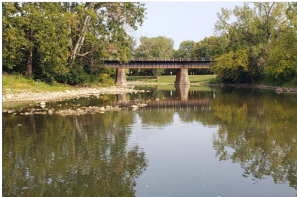
FIGURE 2.8-35 | Former Indiana Steel & Wire dam site following removal September 16, 2020
