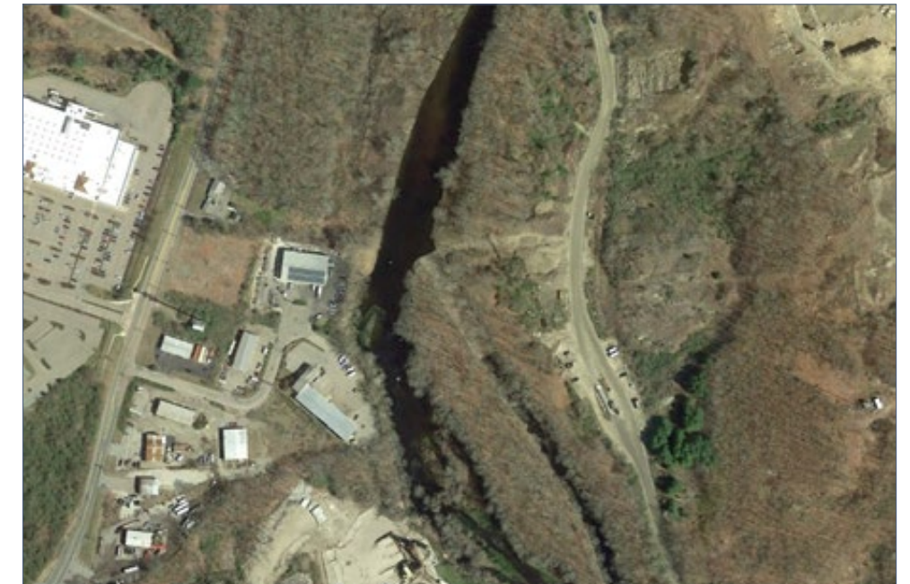
FIGURE 2.8-10 | White Rock Dam after removal, April 2016
