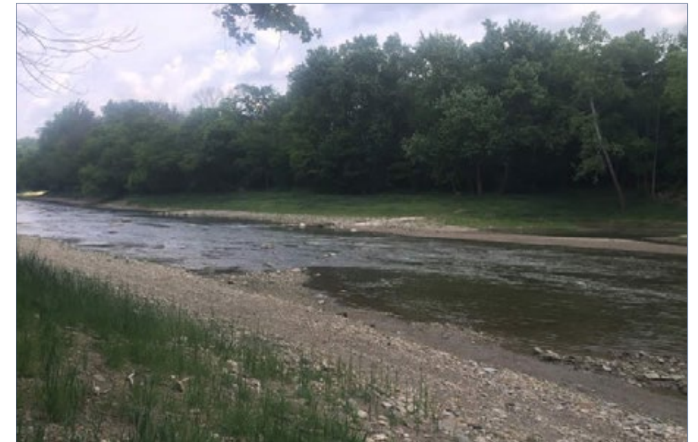
FIGURE 2.8-32 | West Milton Dam after removal
