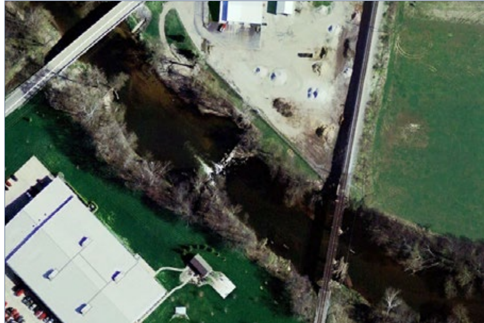
FIGURE 2.8-17 | North Manchester Dam before removal, March 30, 2005
