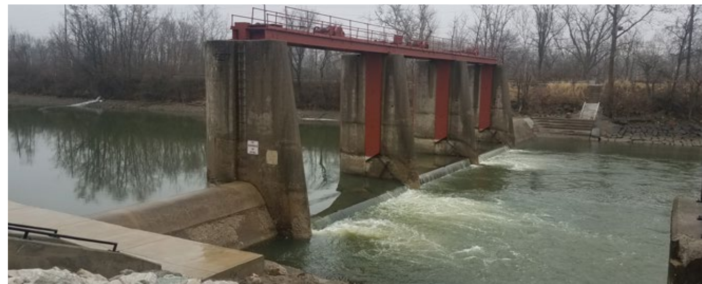
FIGURE 7.2-4 | Existing Condition of the Piqua Power Plant Dam.
