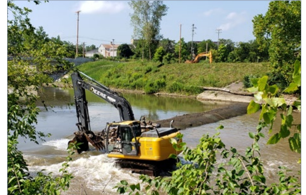
FIGURE 2.8-34 | Indiana Steel & Wire Dam during removal. August 19, 2019
