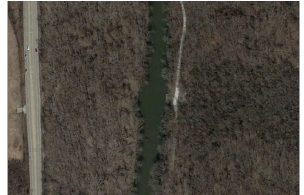
FIGURE 2.8-6 | Armitage Dam after removal.
