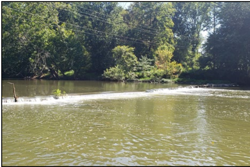
FIGURE 4.6-2 | Piqua Water Company Dam
