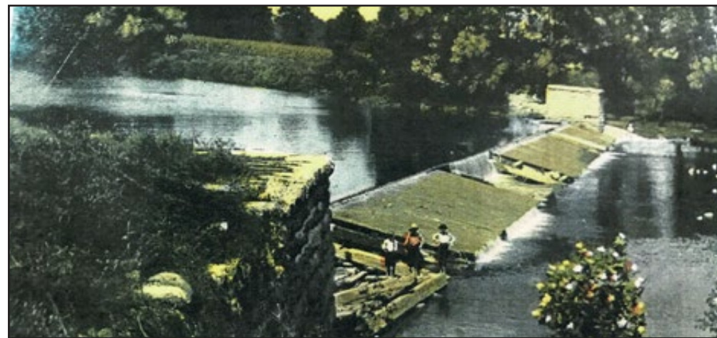
FIGURE 4.5-2 | Original Troy, OH dam (pre 1913). This dam existed between modern-day Treasure Island and Adams St.
