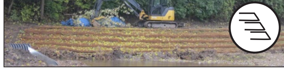
FIGURE 7.4-2 | Vegetated geolift
