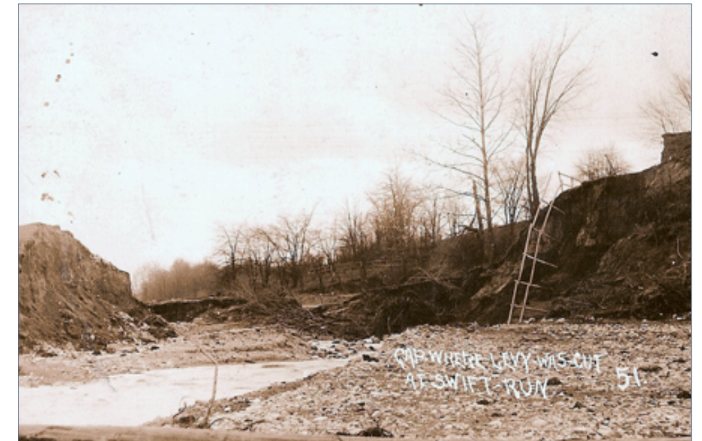
FIGURE 4.4-7 | Gap where the levee was prior to the 1913 flood, Troy, OH
