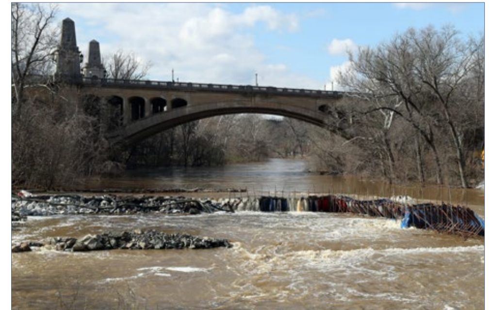
FIGURE 2.8-48 | Water is diverted around a low-head dam in Delaware during removal.
