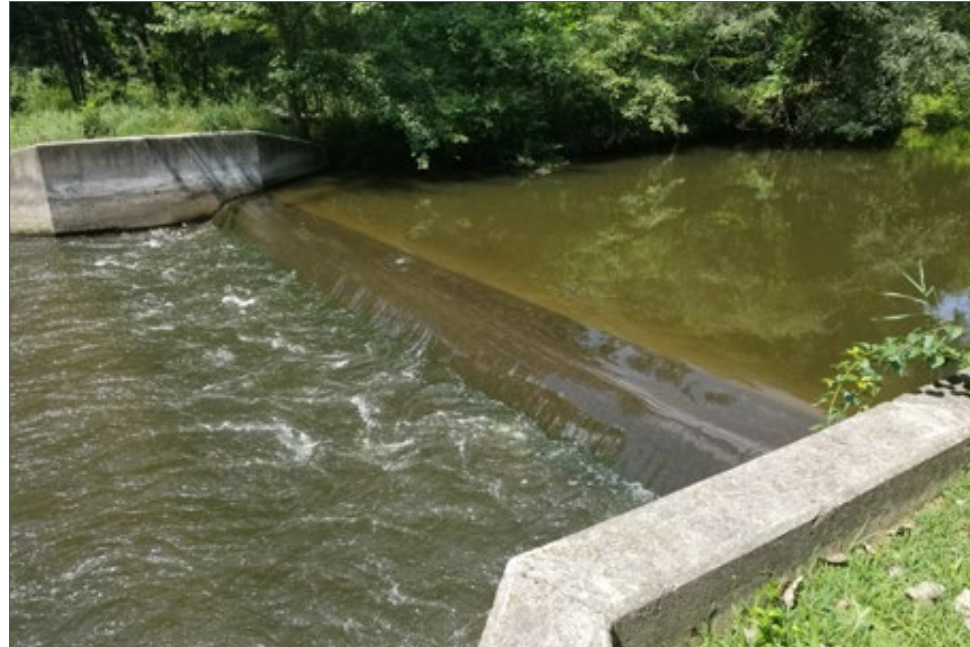
FIGURE 2.8-25 | Fox Farm Road Dam before removal, July 25, 2018
