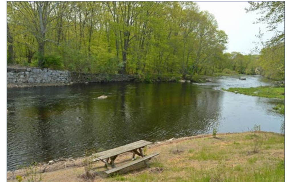
FIGURE 2.8-12 | White Rock Dam after removal
