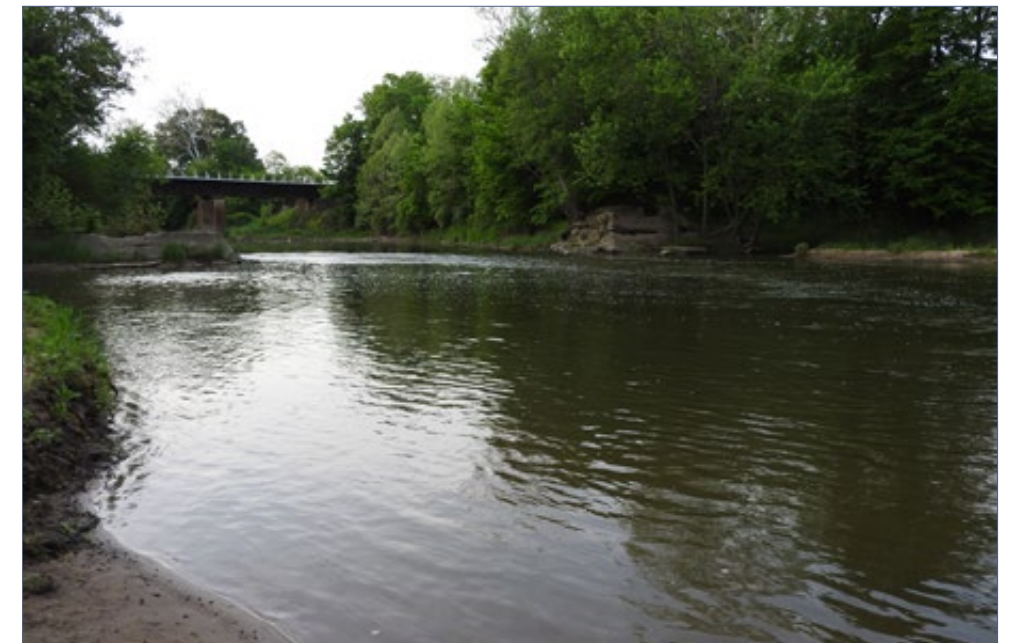
FIGURE 2.8-20 | North Manchester Dam after removal
