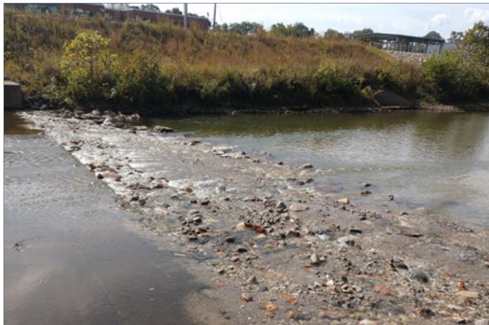
FIGURE 2.8-43 | Completed constructed riffle. October 10, 2019.
