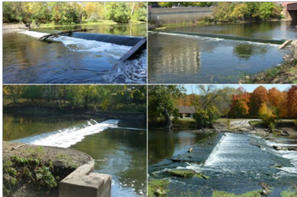
FIGURE 2.8-7 | Armitage Dam before removal.
