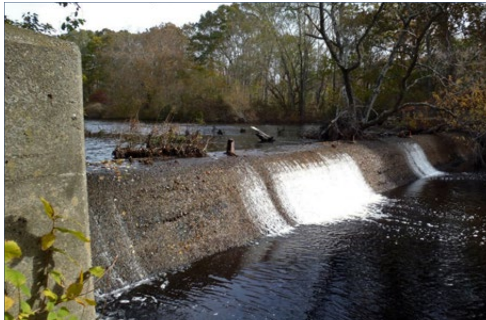
FIGURE 2.8-11 | White Rock Dam before removal
