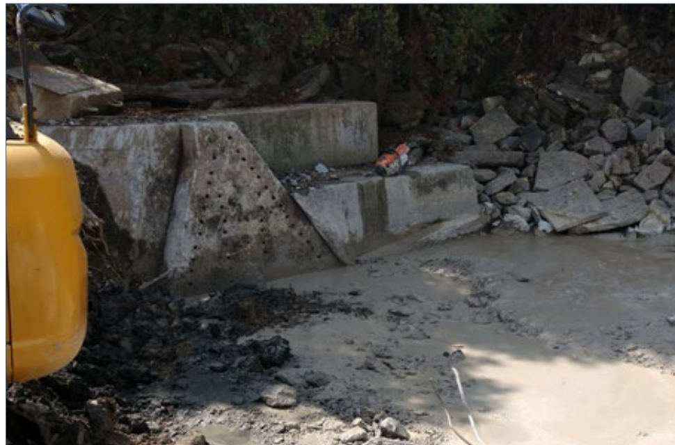
FIGURE 2.8-39 | The ends of the concrete dam were left in place, to maintain stability of the levee toe.
