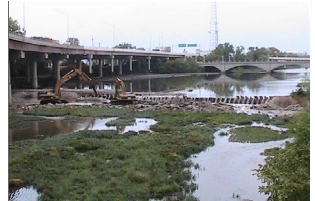
FIGURE 2.8-50 | Removal of the 5th Avenue Dam begins. August 30, 2012.
