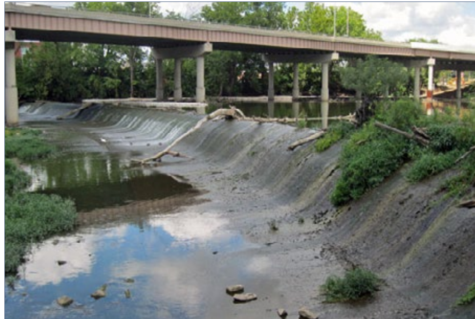
FIGURE 2.8-49 | 5th Avenue Dam before removal, October, 2011.
