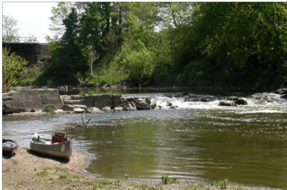
FIGURE 2.8-19 | North Manchester Dam before removal.
