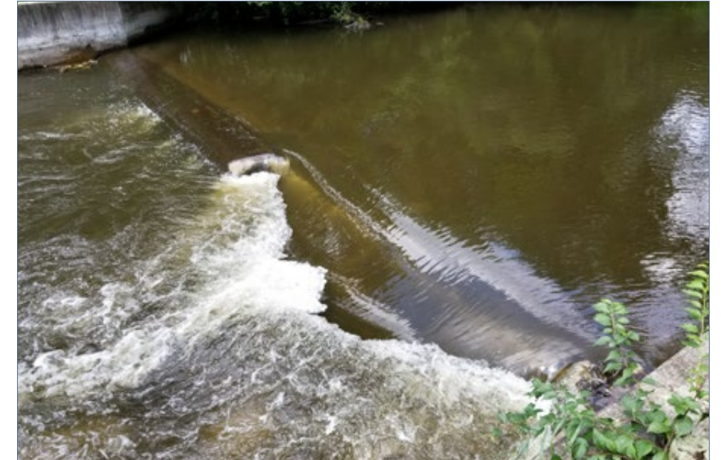
FIGURE 2.8-26 | Initial dam breach during removal process. August 10, 2018.
