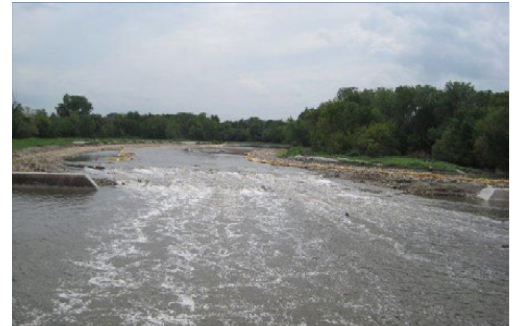
FIGURE 2.8-4 | Hofmann Dam after removal
