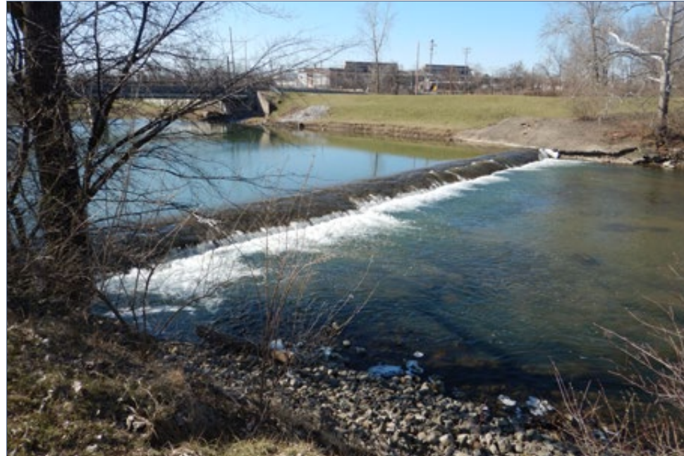
FIGURE 2.8-33 | Indiana Steel & Wire Dam before removal. March 16, 2017
