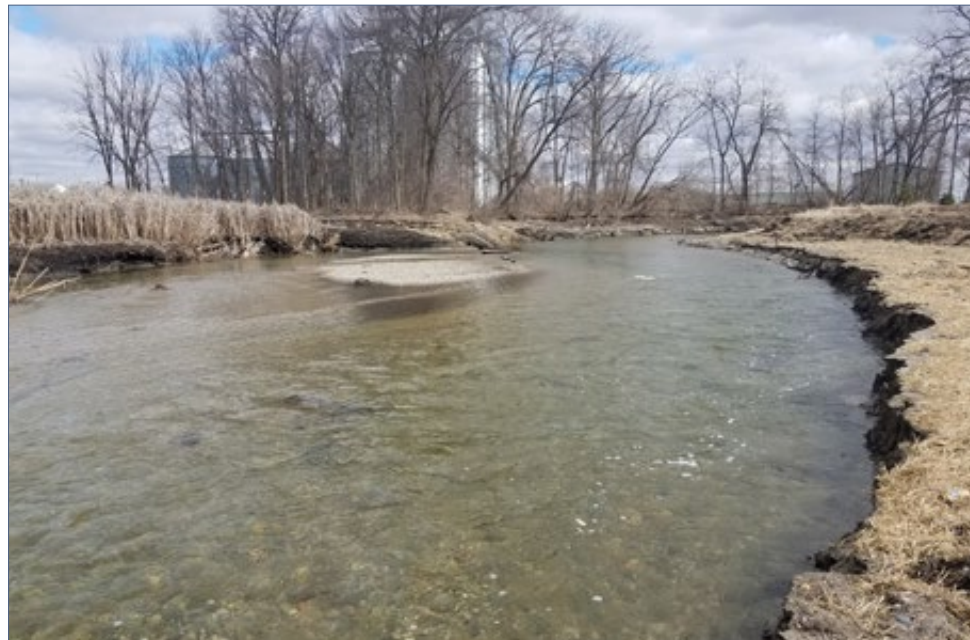
FIGURE 2.8-23 | Former backwater of the Fawn River Dam, following removal, March 15, 2018.
