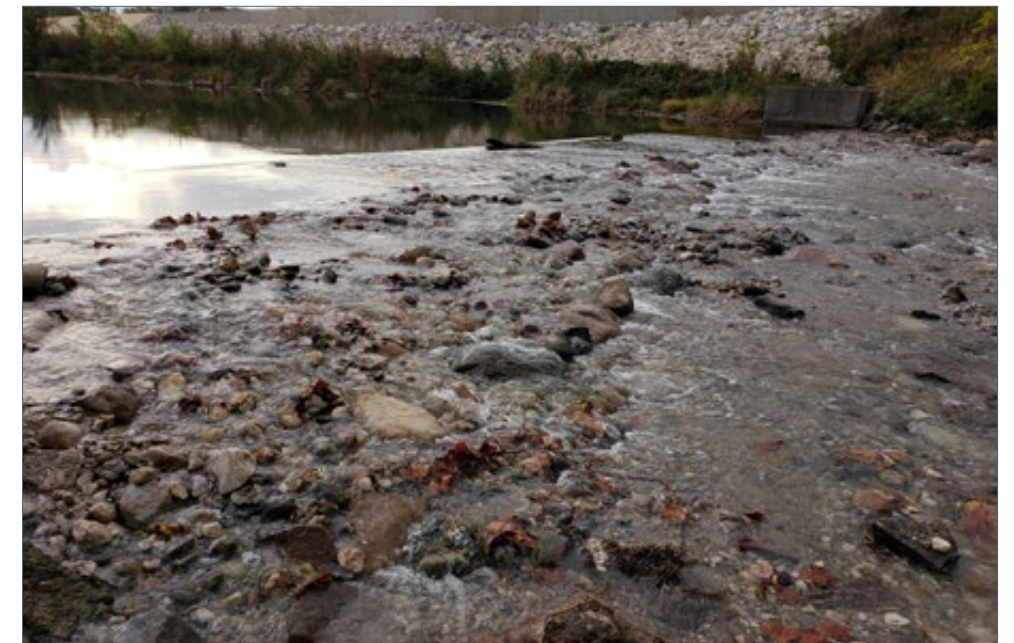
FIGURE 2.8-44 | Completed constructed riffle. October 11, 2019.
