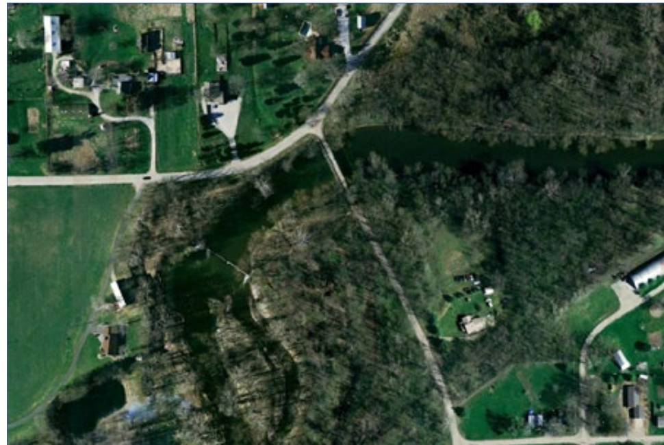
FIGURE 2.8-13 | Liberty Mills Dam before removal, March 12, 2012
