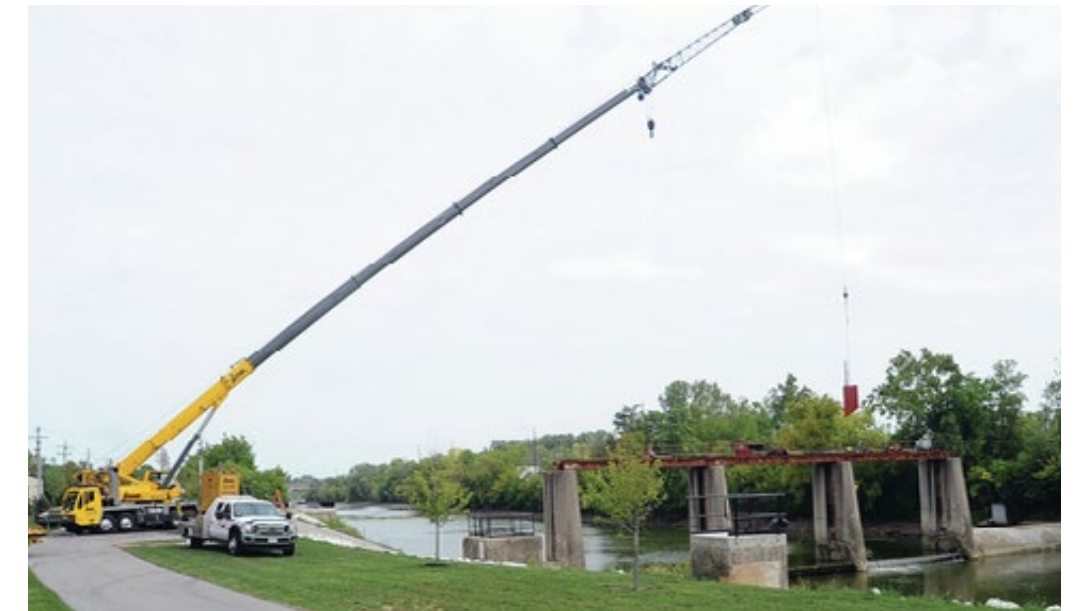
FIGURE 7.1-1 | A large crane makes repairs to the dam's adjustable gates.
