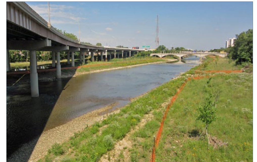
FIGURE 2.8-52 | Former Site of the 5th Avenue dam following restoration.
