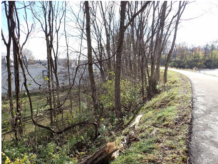
5. A view of the downstream slope at the left end of the dam. Note the trees and heavy brush.
