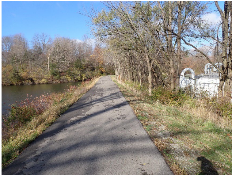
4. A view of the crest of the dam.
