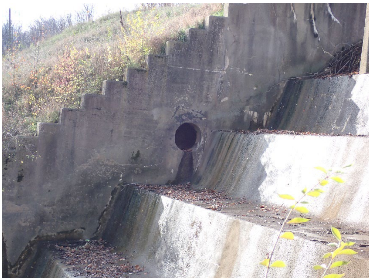
21. The lake drain discharges through the right sidewall of spillway #3.
