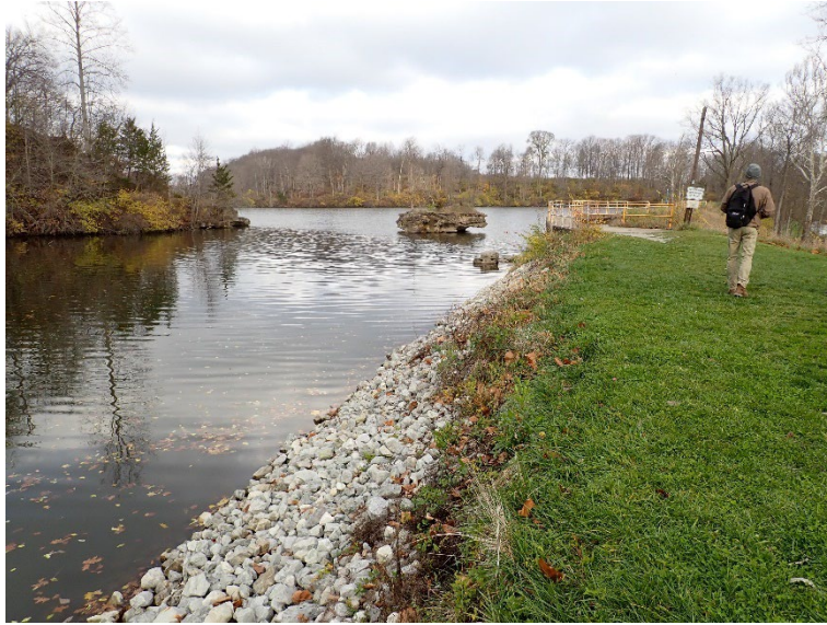
1. Upstream slope and crest at the far-right end of the dam.
