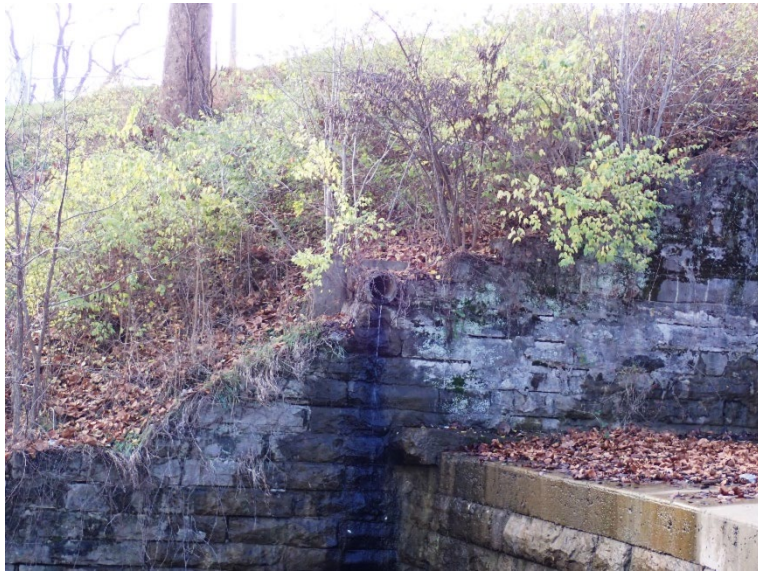
10. Downstream slope to the right of spillway #2. Note trees and dense overgrowth of brush.
