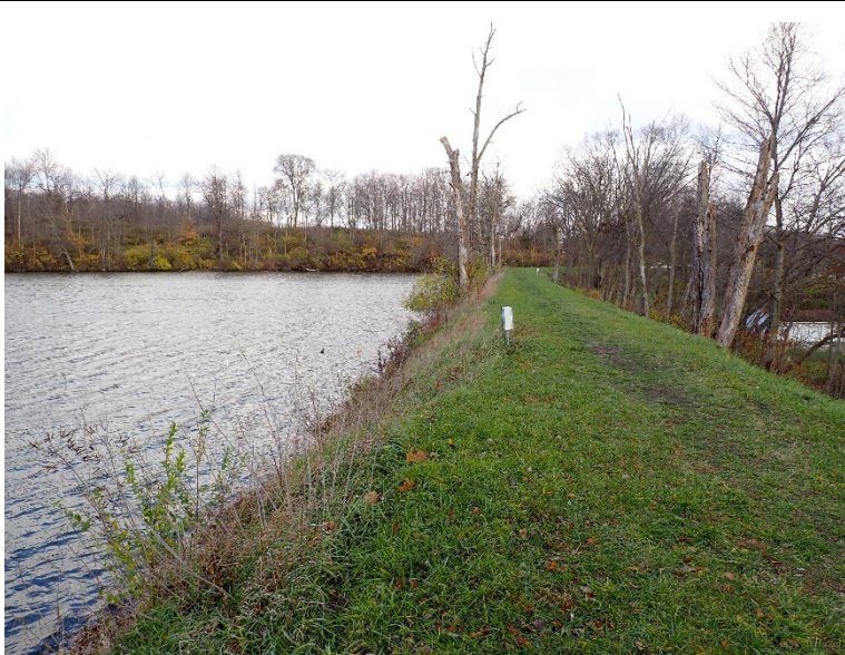
4. Upstream slope and crest to the left of spillway #3.
