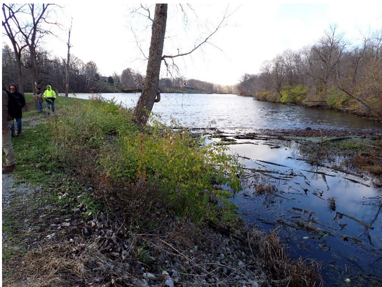
6. Upstream slope at the far-left end of the dam. Again, note the tree and the too tall vegetation.
