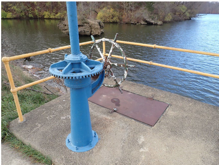
17. Lake drain control at the right side of spillway #3.
