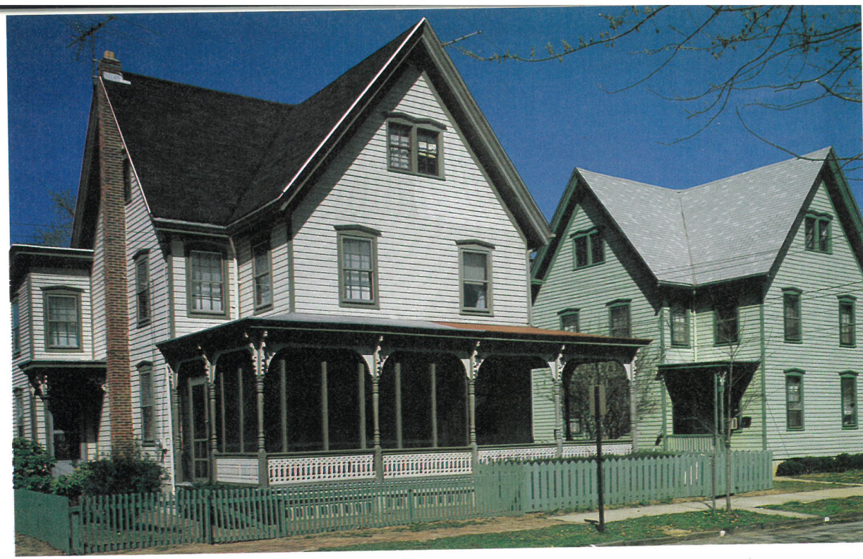
PLATE 6. Modest Victorian houses of no particular style are found in historic districts across America. Here the four owners of twin houses cooperated in color selection, assisted by a representative of the local housing office charged with enforcing the color clause in the historic-district zoning ordinance. The house on the left has a Light Drab body, Dark Drab trim, and Reddish Brown sash. The house on the right has a Light Blue Green body with trim in Dark Blue Stone and sash painted in Shutter Green. (The unfortunate color change in the gable of the house on the left resulted from two weekend painters working from two cans of the same brand and color of paint on different weekends. Had a single painter started at the top and worked across the entire gable, such differences, which can occur even when painting with seemingly identical colors, would not have been so obvious.)
